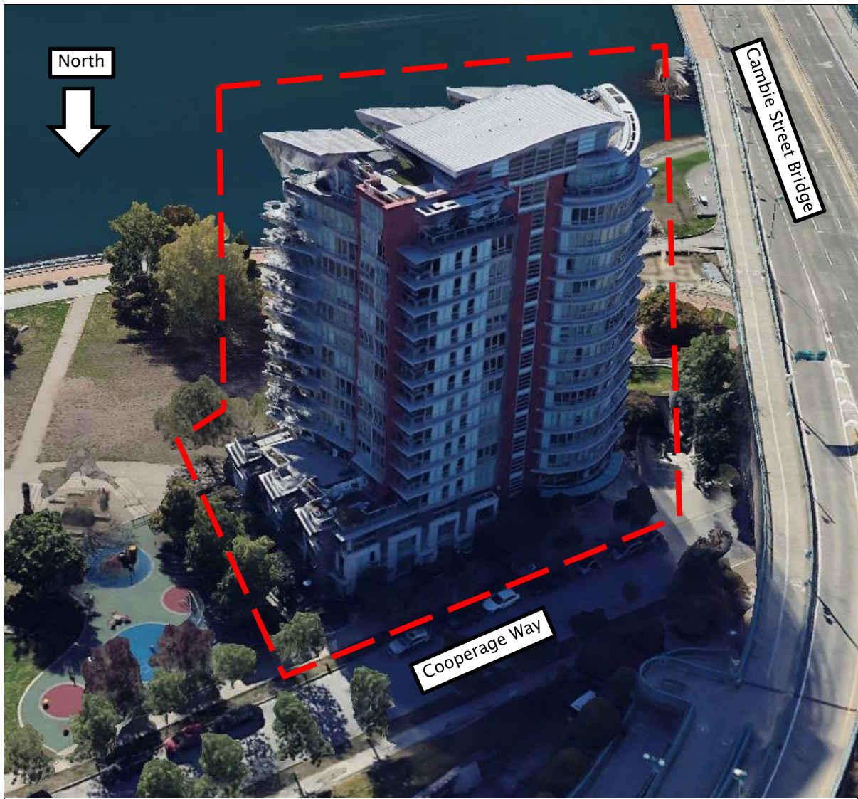
Figure 2.2 Aerial photograph of Coopers Pointe (©Google 2024).
